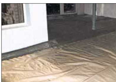
Installation of separating layer
