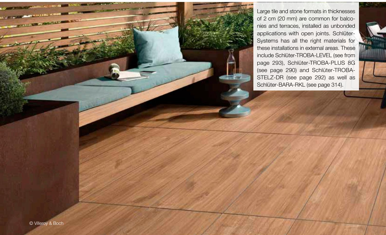
Large tile and stone formats in thicknesses of 2 cm (20 mm) are common for balconies and terraces, installed as unbonded applications with open joints. Schlüter-Systems has all the right materials for these installations in external areas. These include Schlüter-TROBA-LEVEL (see from page 293), Schlüter-TROBA-PLUS 8G (see page 290) and Schlüter-TROBA-STELZ-DR (see page 292) as well as Schlüter-BARA-RKL (see page 314).
