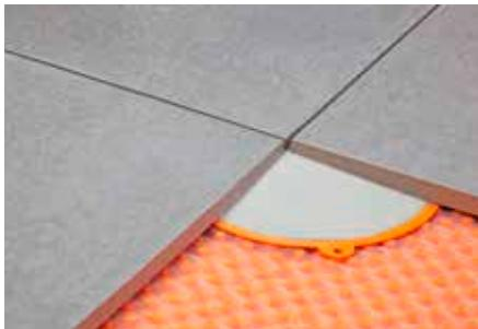
Schlüter-TROBA-STELZ-DR are formwork rings for thin bed mortar installed over Schlüter-TROBA-PLUS. After the installation of mortar, the rings can either remain in place or be removed and reused.
