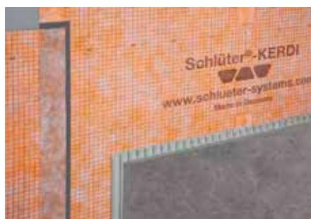
Schlüter-KERDI is a polyethylene waterproofing membrane with an anchoring fleece laminated on both sides. It is suitable for waterproofing in conjunction with tiled surfaces on walls and floors. The high water vapour diffusion resistance of Schlüter-KERDI-DS makes it suitable as a vapour barrier in bonded floor assemblies with tile coverings.
