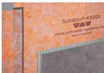
Schlüter-KERDI is a polyethylene waterproofing membrane with an anchoring fleece laminated on both sides. It is particularly well suited for outdoor waterproofing below surface drainage assemblies with Schlüter-TROBA-PLUS or bonded drainage assemblies with Schlüter-DITRA-DRAIN.
